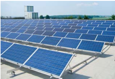
Mounting directly in concrete roof
